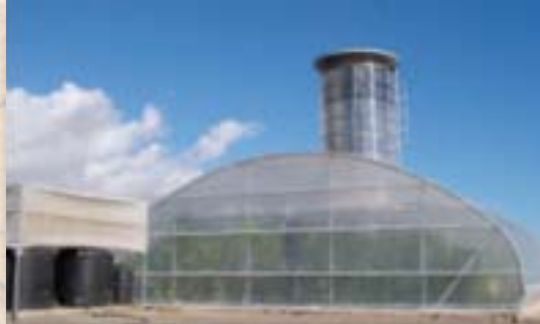
Mr. Martin Buchhloz is the author of Watergy prototype greenhouse built in Almería, Spain (photo), as well as the patent. Next to reduction of costs in space cooling and heating, the system can be fed with waste water to obtain distilled water.
